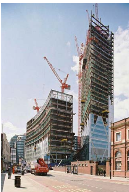
Progress picture April 2007
